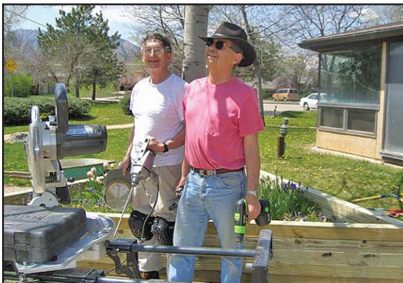
DON LILLEY AND REED BAILEY REPLACING WOODEN PLANTER FRAMES (CIRCA 2006)
