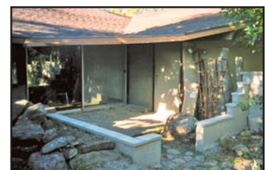
REMOVING INTERNAL GARDEN WALLS, CIRCA 2000
